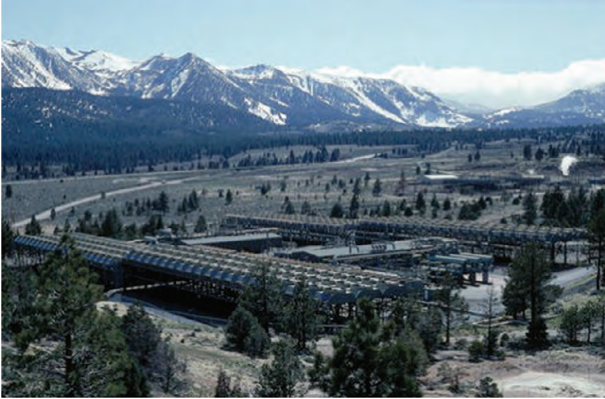
Figure 13. Air-cooled binary plants near Mammoth Lakes, California
