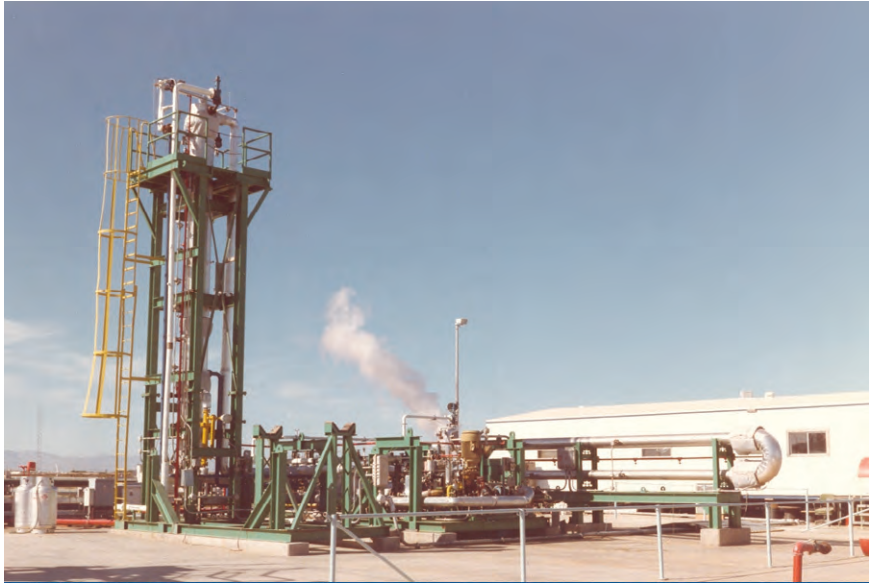
Figure 25. Heat Cycle Research Facility with a vertical condenser orientation
