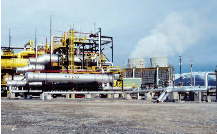
Figure 3. Raft River 5-MW binary pilot plant, Idaho
