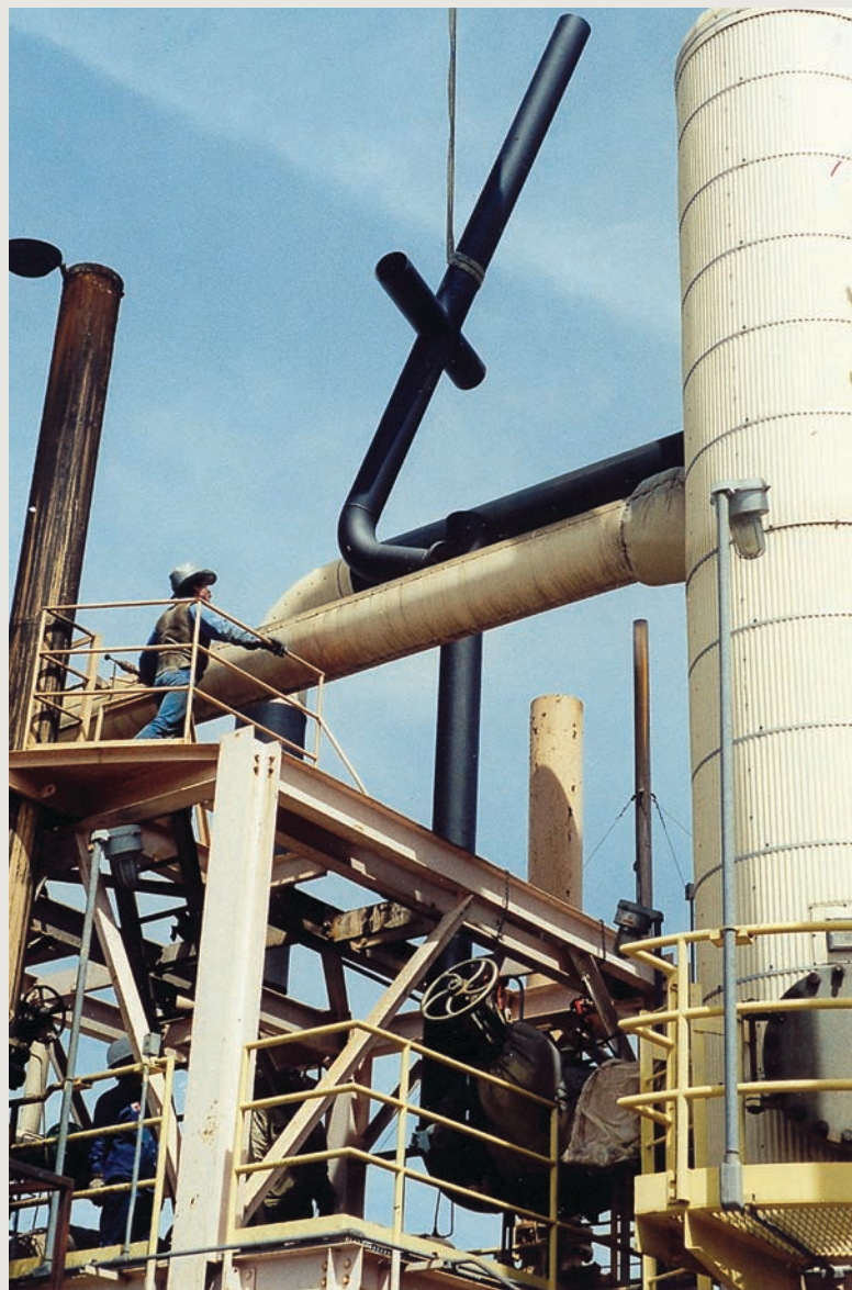
Installation of a PPS-coated steam vent at Cove Fort in Utah.
