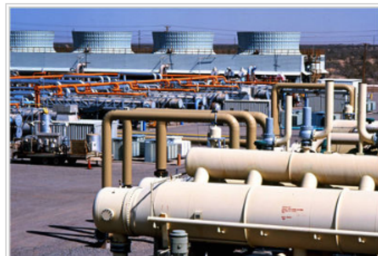
Binary power system equipment and cooling towers at the ORMAT Ormesa Geothermal Power Complex in Southern California. [edit]
