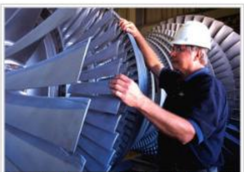
An engineer inspects the blades of a backup turbine at a Northern California Power Agency (NCPA) geothermal power plant at The Geysers.
