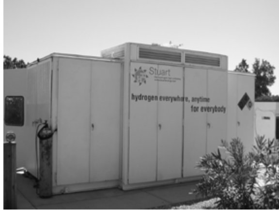
Figure 4. Stuart Energy's modular compressed hydrogen station
