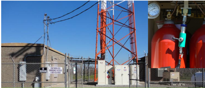
Refueling hydrogen tanks for backup power (top right); AT&T cellular tower site with fuel cells for backup power. ReliOn, Inc.
