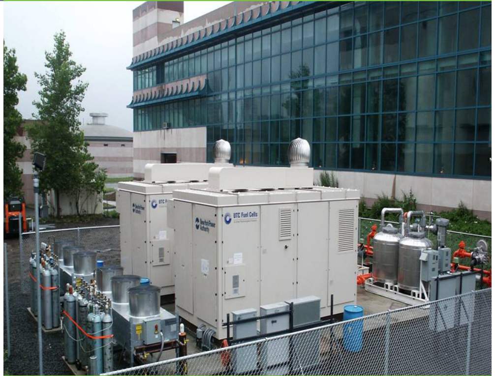
Fuel cells in a combined heat and power installation. Courtesy of UTC Fuel Cells.
