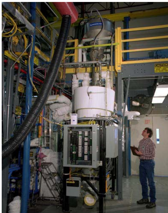
Figure 2: Fluid bed reformer installed in NREL TCUF
