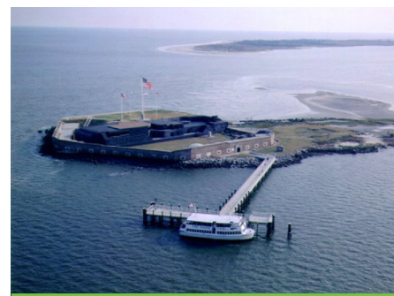
Fuel cell backup power at Fort Sumter National Monument in South Carolina.
