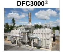
**Co-product** Power, kW 250 1,000 2,000 Hydrogen, kg/day 125 500 1,000 0.5 2.0 4.0 Heat, mmBtu/hr **Peaker Capacity** Peak Power (8 hrs/day), kw **500** 2,000 4,000 **Refueling Capacity** Fuel Cell Cars, 0.5 kg/day 300 1,200 2,400
