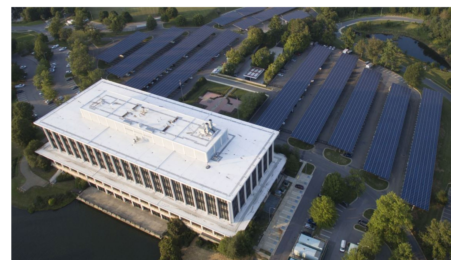
Microgrid installed (2020) at the Montgomery County Public Safety Headquarters in Gaithersburg, MD. The project includes 2 MW of solar PV and an 800 kW CHP system (Credit: Montgomery County, MD)
