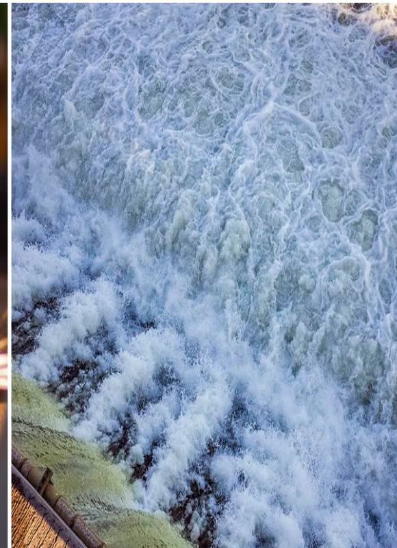
Water & Wastewater Treatment
