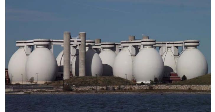
Deer Island Wastewater Treatment Plant in Boston
