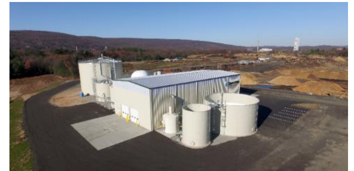
Quantum Biopower Food Waste Digester in Connecticut
