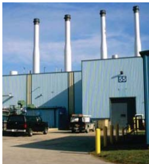
SC Johnson Cogeneration Facility
