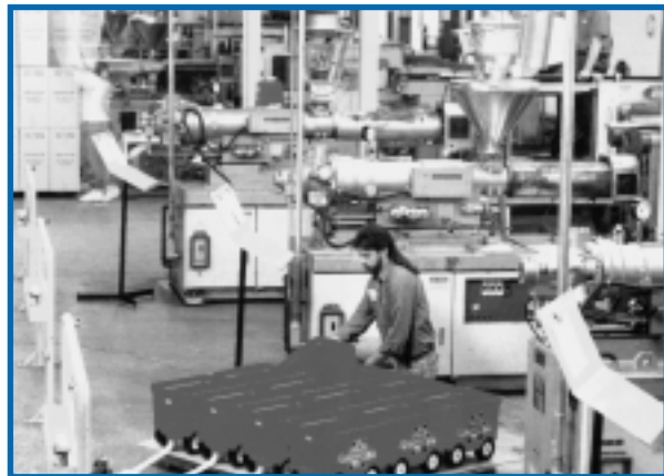
Highland's molding machines benefitted from a VFD retrofit.
