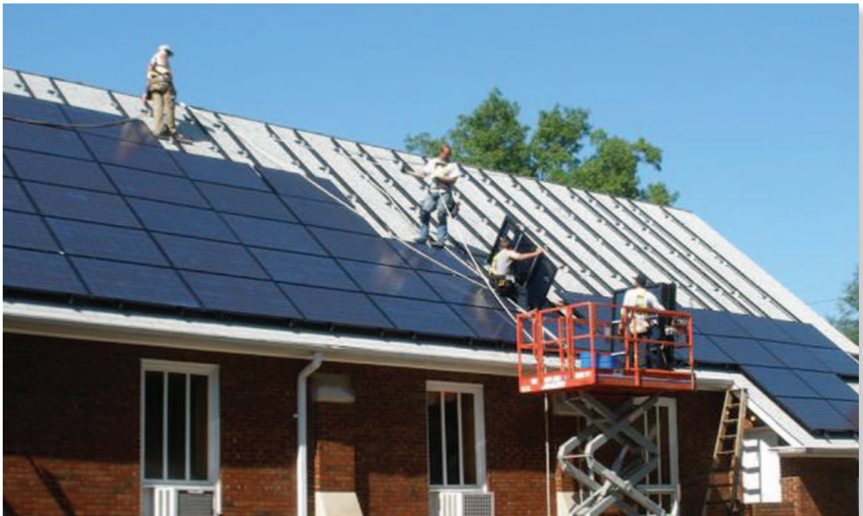
Installing Panels on the Church of the Bretheren, University Park, Maryland
