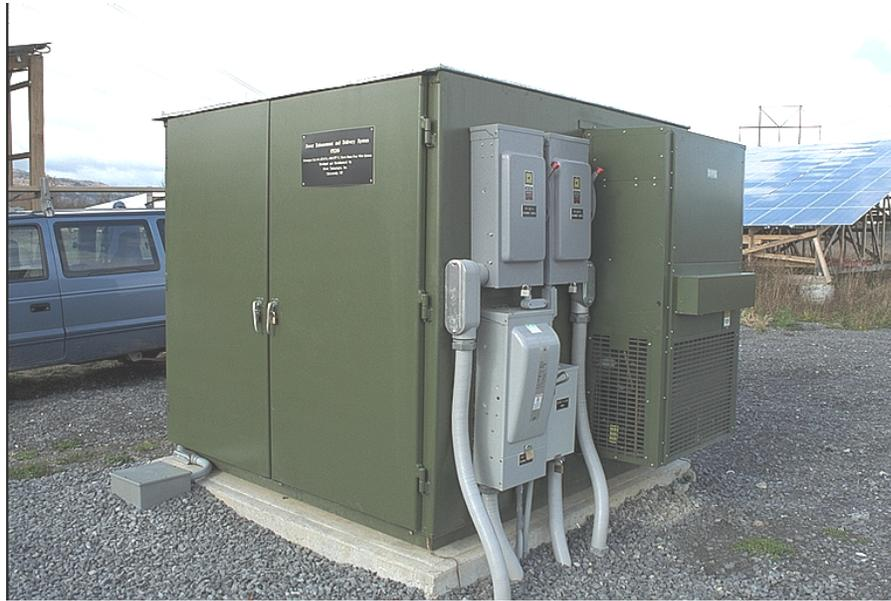
**Figure B-7. Example of a 125-kW PV UPS unit developed by Power Technologies, Inc., for Niagara Mohawk Power Corporation in the late 1990s**
