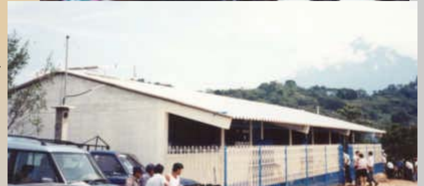
Students enjoy their first distance education class with a newly-installed PV system in rural Guatemala
