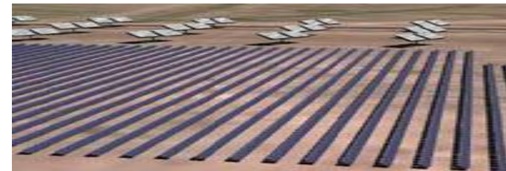
8MW PV Plant, Alamosa, CO
