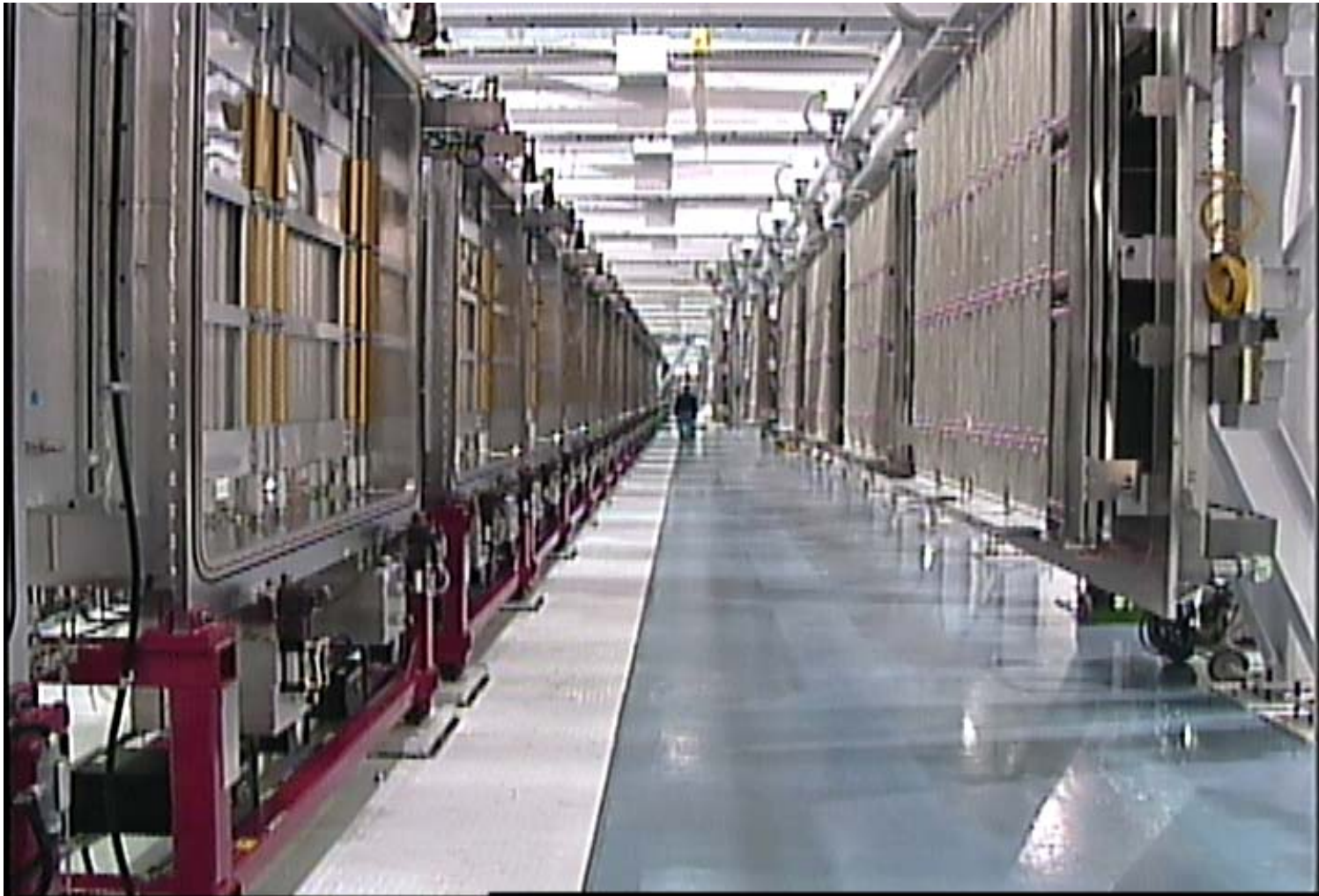
30MW Machine – Chambers (L) Doors (R)
