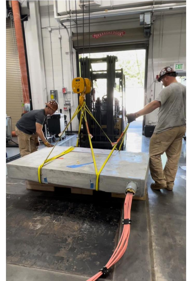
200 kW DWPT system with transmitter set in precast Master flow 648 Epoxy Resin Grout
