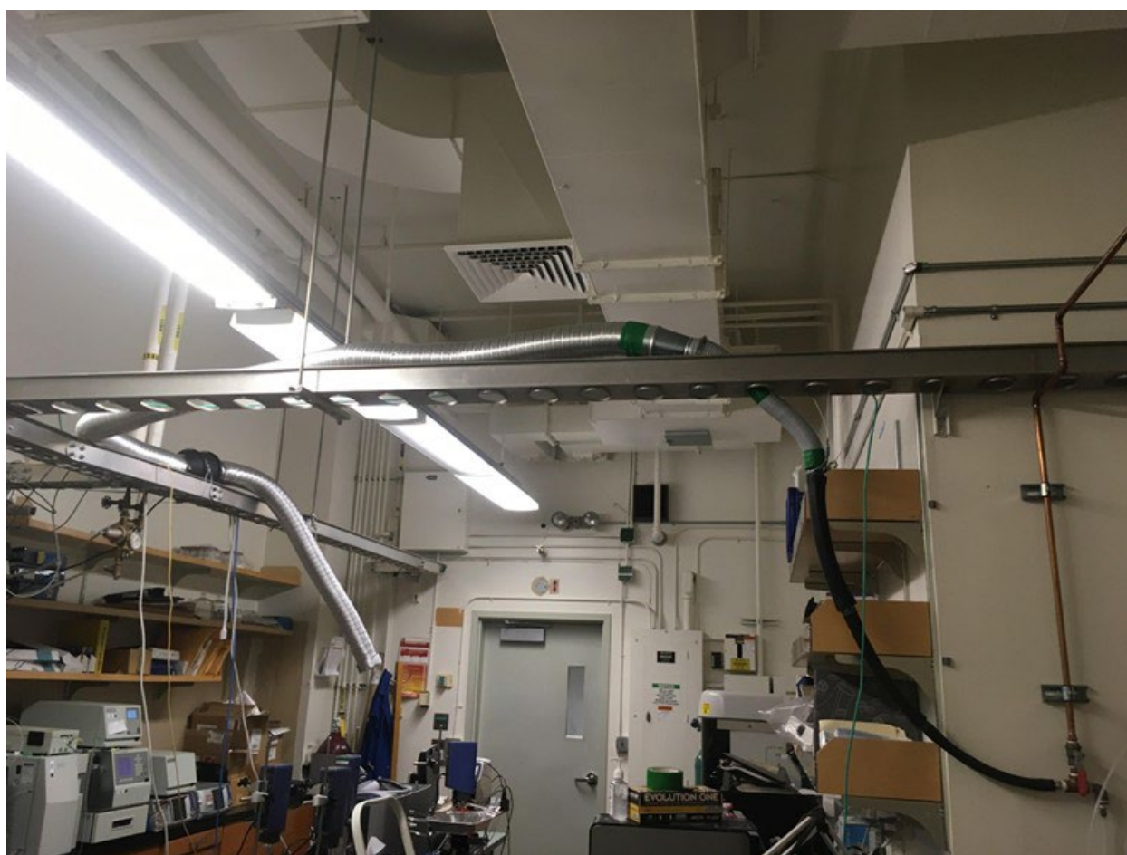
Figure II.6.1 Vapor extraction system (K. Higa/LBNL)
