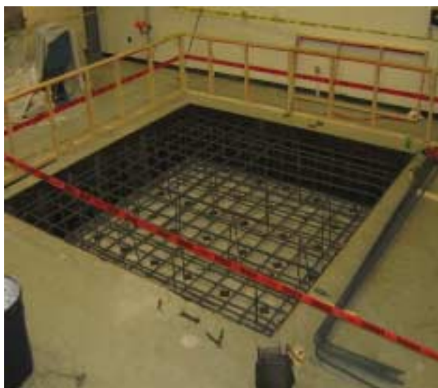
Figure 4. Site preparation for press installation.
