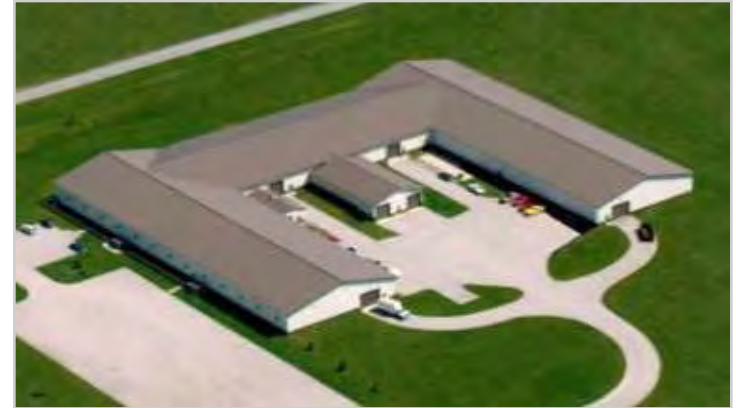
Delphi's Power Electronics Manufacturing Site Kokomo, Indiana
