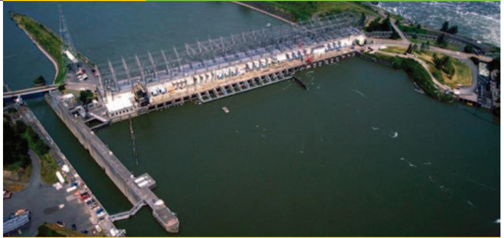
The Bonneville Dam on the Columbia River between Washington and Oregon has 20 turbines with a total capacity rating of more than 1,000 megawatts. Courtesy of the U.S. Army Corps of Engineers
