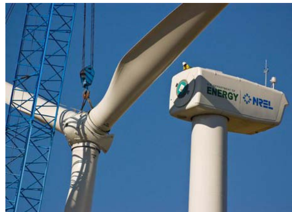
Figure 10. Installation of DOE 1.5 MW turbine
