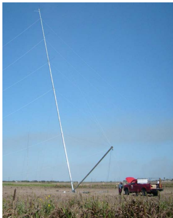
Figure 59. Meteorological tower installed at GSA facility in Texas
